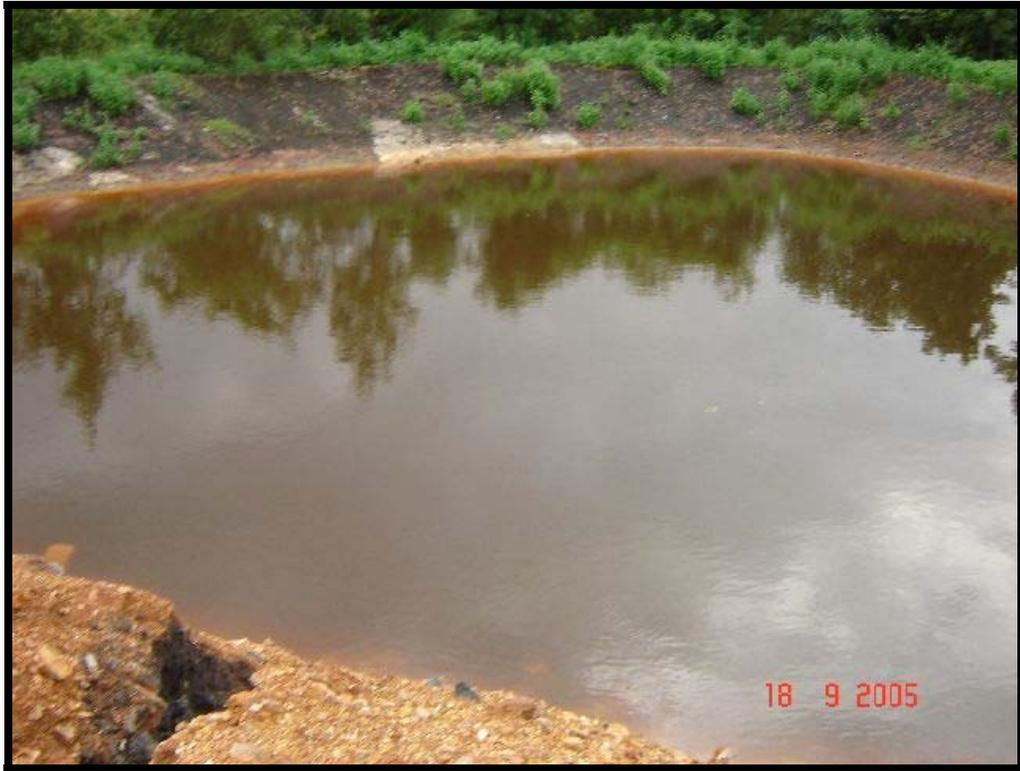
P.N. The Dyke of the Slush pond is cracked and the untreated pond water flows out into nearby nallahs and low lying land areas
