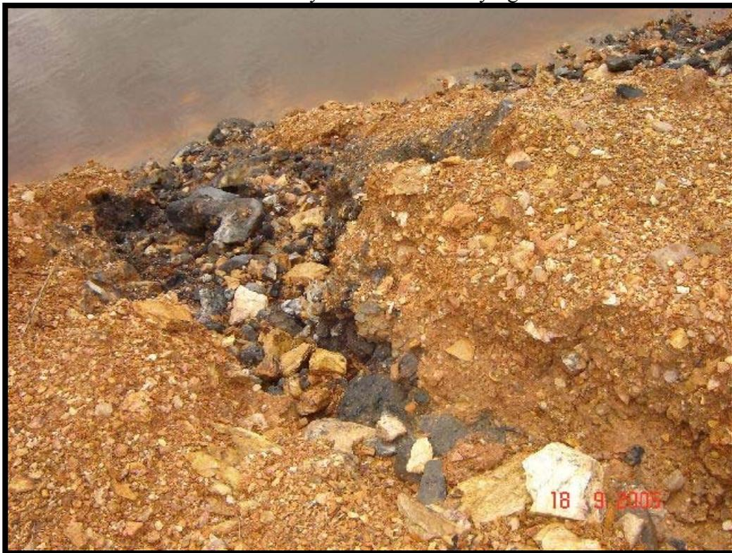
P.N. The Slush pond has not been provided with polythene lining so the pond water constantly leaches out from the bottom and sides of the pond.
